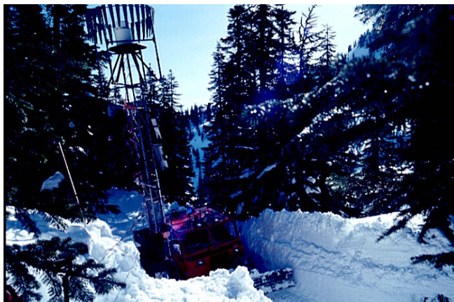
Figure 2. The overburden pressure of a very deep snowpack on this tower's guy wires pulled it off vertical over the course of a month or two. Photo courtesy Mark Moore.
