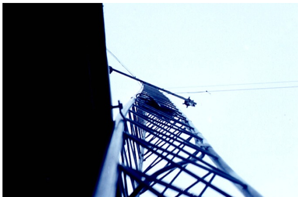
Figure 1. The weight of snow on the guy wires for this tower at Hurricane Ridge in the Olympic Mountains of Washington State bent the legs of this tower, resulting in an expensive replacement. Mark Moore photo.
